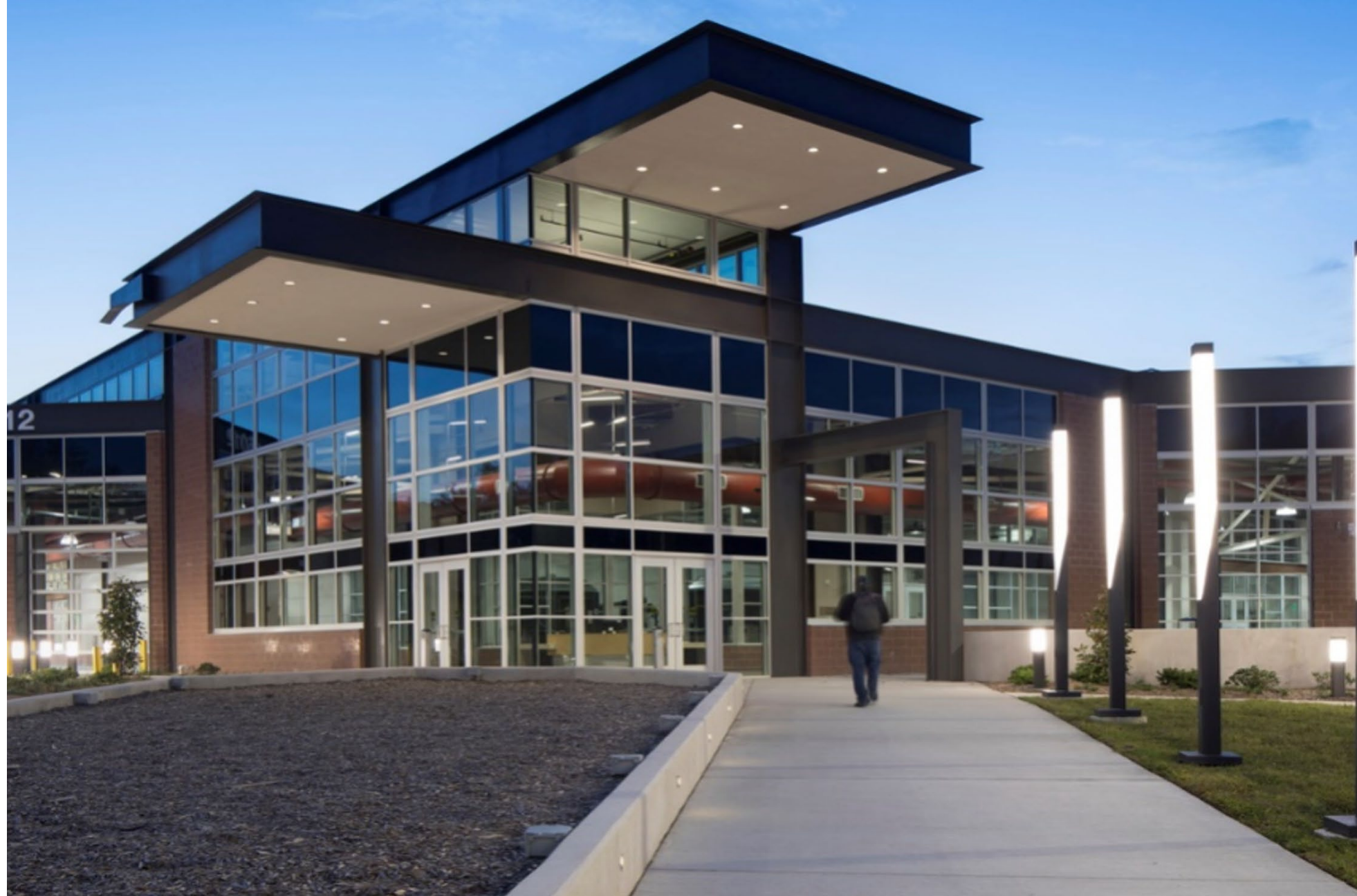
Guilford Technical Community College—Center for Advanced Manufacturing
